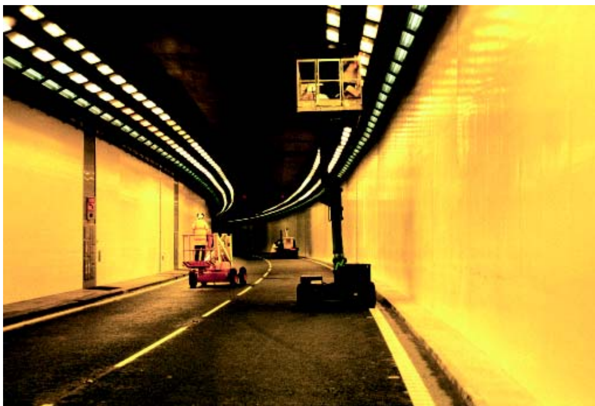
Figure 8. 1: Cleaning the Luminaires
