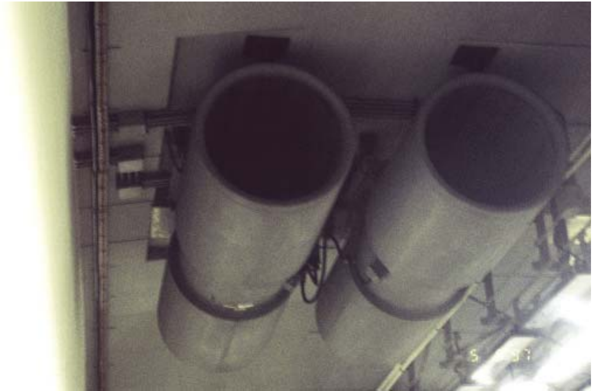
Figure 7.1: Jet Fans providing Longitudinal Ventilation
