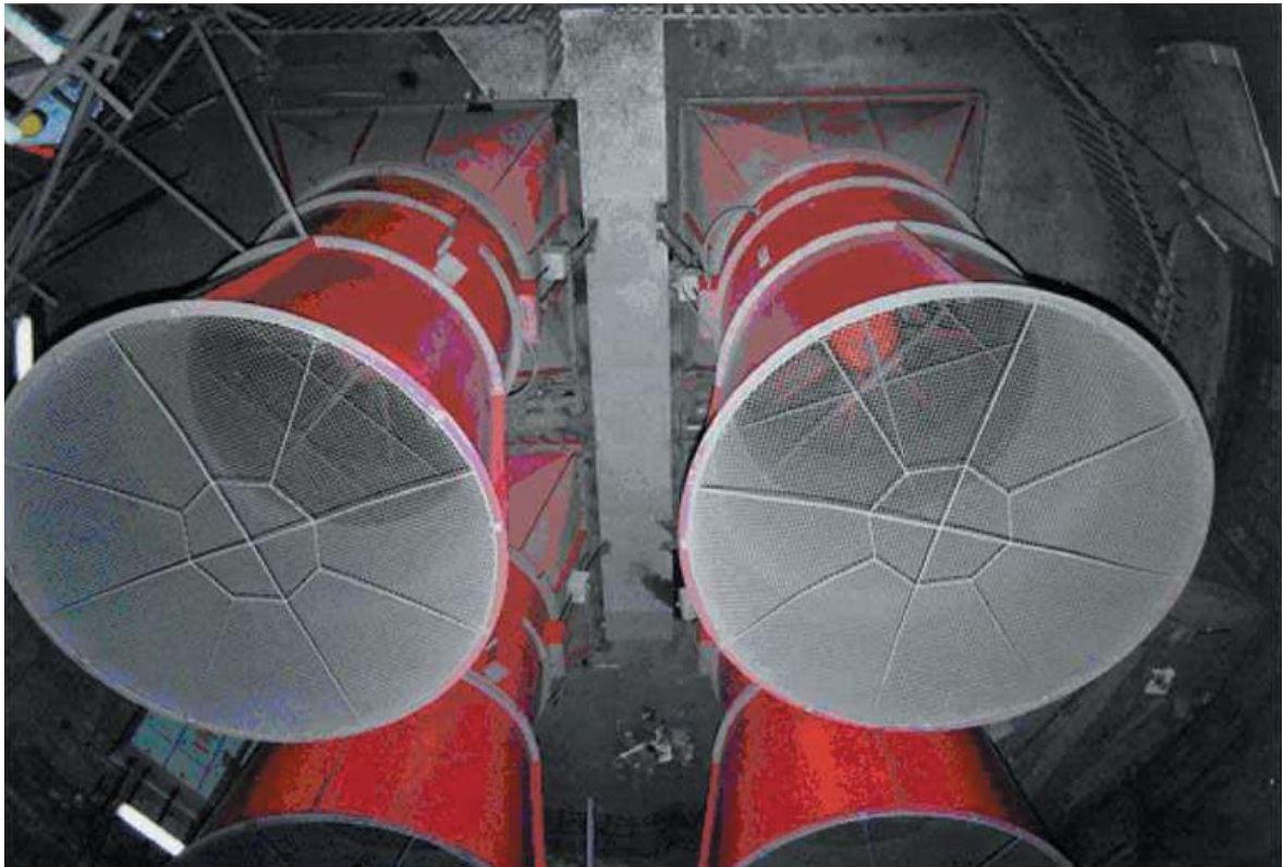
Figure 7.2: Fixed Axial Fans over Supply/Extract Shaft
