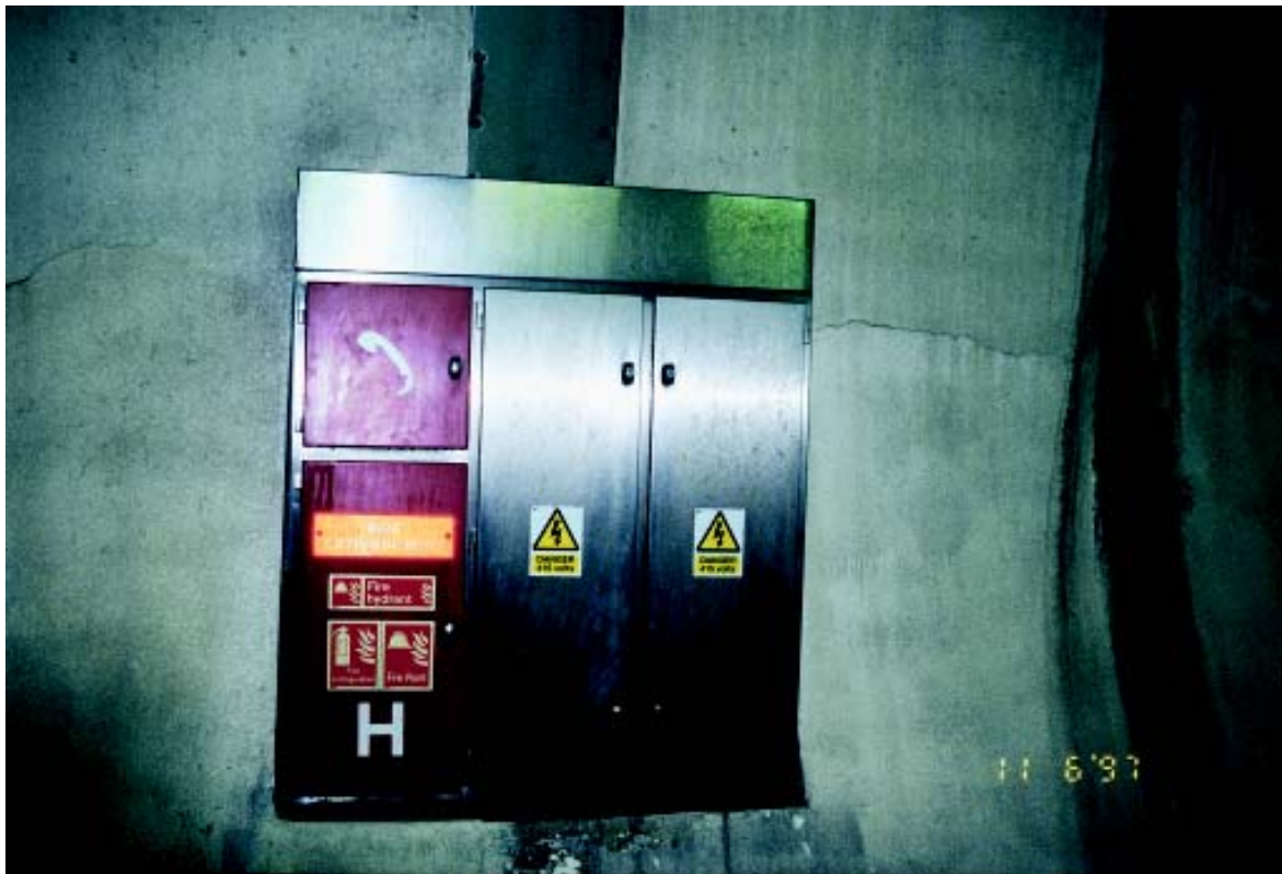
Figure 10.1: Tunnel Emergency Panel
