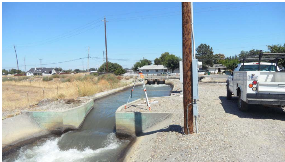
Figure 53. Example of a poor installation site: upstream is a control gate; downstream is a drop in elevation with turbulent flow
