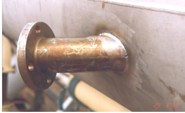
Figure 13: Transducer holder welded to the pipe.
