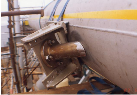
Figure 12: Welding jig and transducer holder.
