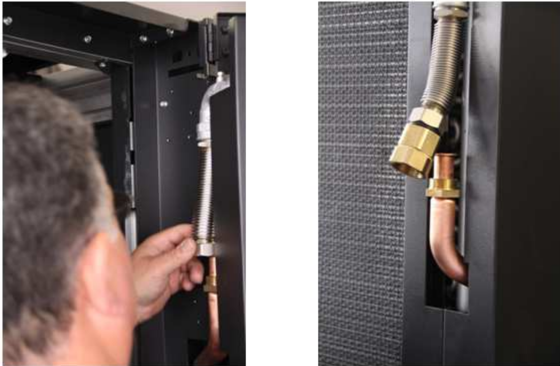
Fig. 16 Flexible piping
