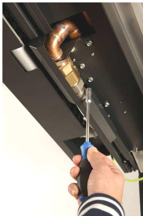
Fig. 22 Attaching the swivel joint covers
