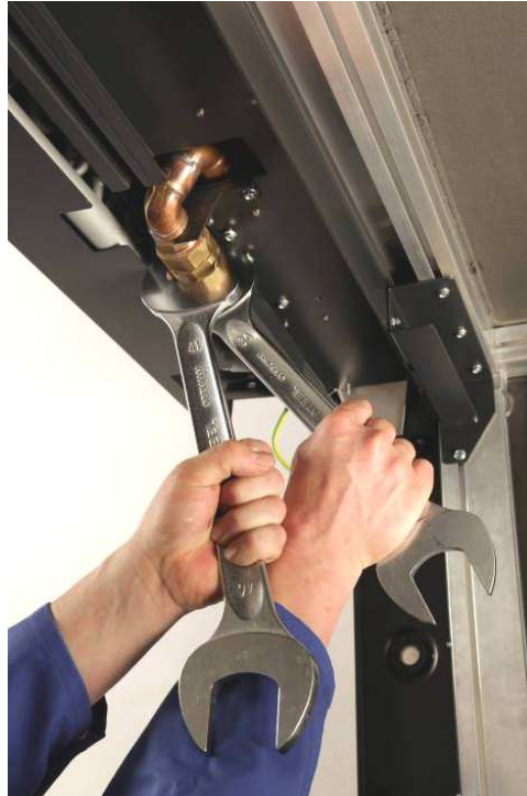
Fig. 18 Tightening the union nuts
