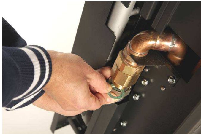
Fig. 17 Inserting sealing rings
