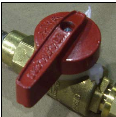
Step 2. Shut off gas valve at appliance.
