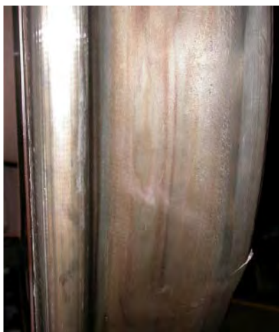
Photograph 9 Sub surface fatigue crack Note: protrusion on chamfer/rim of wheel
