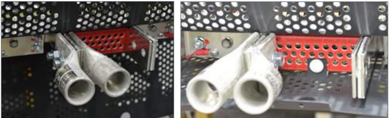
Figure 13 — Lug Connection, middle push-clip
