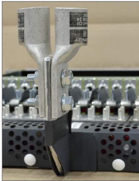
Figure 17 — Lugs Mounted to Vertical Adapter
