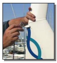
Attach the recovery lanyard to the shackle on the yaw arm. Form a loop on the inboard end and drop it over the hook on the upper tower clamp.
