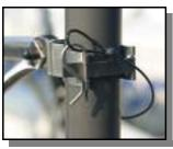
Check that the top tower bracket strap is securely closed and that the locking pin is in place (see box left). Check that the alternator yoke is locked centrally by tightening the thumbscrew. Orientate the yaw arm so that you will be fitting the turbine downwind, and ensure that it remains downwind throughout the operation.
