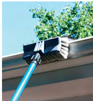
Cleaning Gutter Exterior
