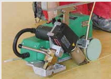
Step 2: Inserting the welding rod into the groove with the UNIFLOOR E hot-air welder.
