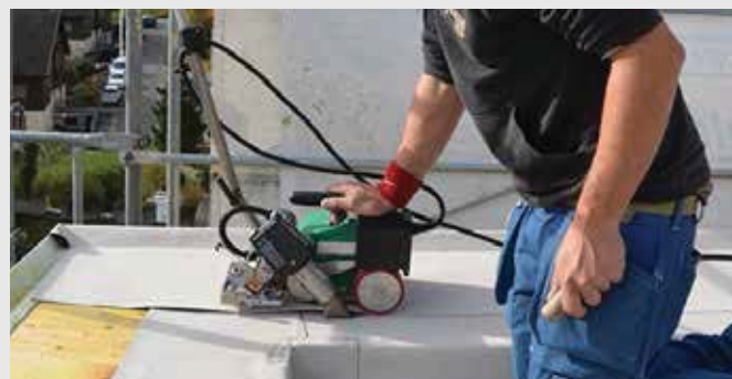
Clean overlap welding of base welds.
