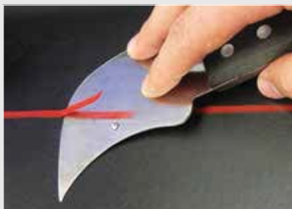
Step 4: Leveling the protruding welding rod with the spatula.
