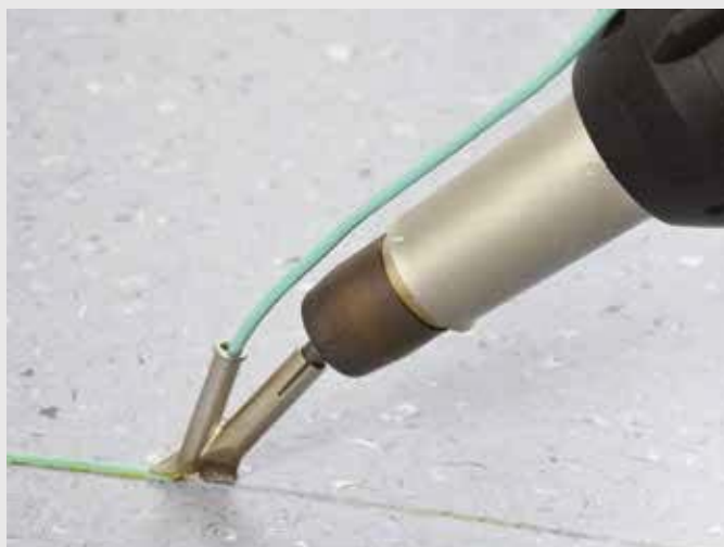
Step 4: Leveling the protruding welding rod with the spatula.
