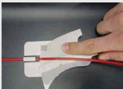
Step 3: Remove the excess welding rod with trimmer guide and spatula
