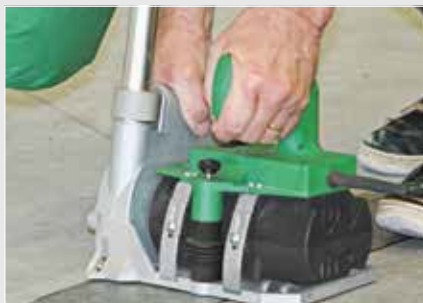
Step 1: Milling the groove with the GROOVER.
