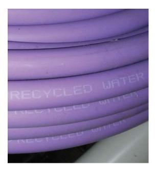
All pipes or pipe sleeves and identification tapes (including those on greywater irrigation systems) shall be coloured purple as per AS 2700 and marked with the following in accordance with AS 1345 "WARNING RECYCLED WATER – DO NOT DRINK" at intervals not exceeding 0.5 m.
