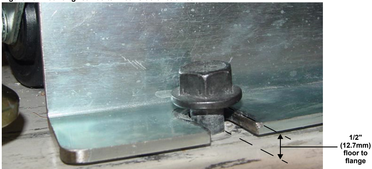
Figure 13 Mounting rear bolts—rear side of cabinet
