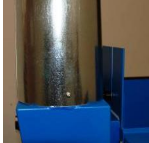
Figure 11. Secure Exhaust Ventilation Stack
