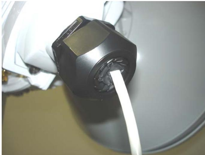
Figure 30 Cord Grip Tightened (Single Cable Install)
