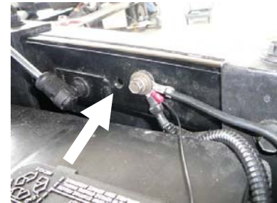
Ground connector installed: Part 1C
