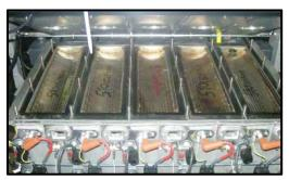
Figure 7-23: Burner Modules Exposed for Cleaning
