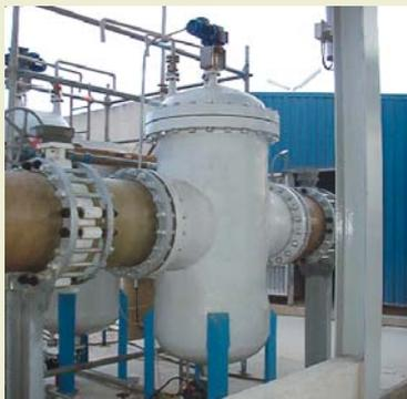
Large size filters designed to suit specific industrial needs, made out of carbon steel, plastic materials, stainless steel or any other material or alloy required by your process. A complete range of filtering elements with different styles and made out of various materials. Painting or coating cycles based on the operation environment. Everything required to offer an accurate and reliable filtering service.
