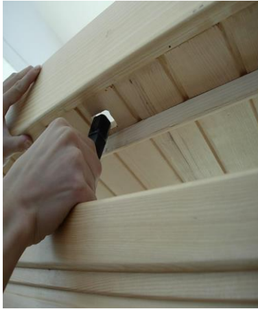
FIG 12 Slip cords/wires through corresponding holes
