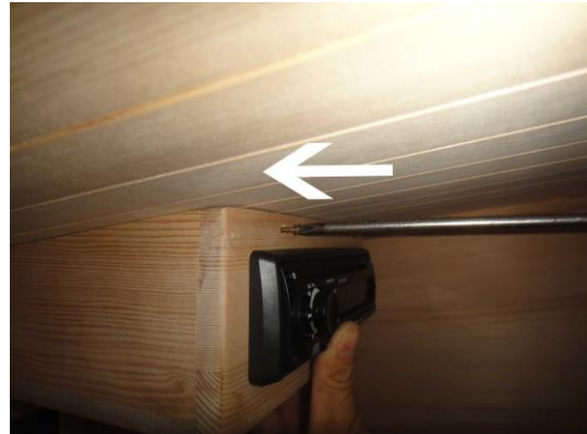
FIG 15.4 Screw wood housing to sauna room
