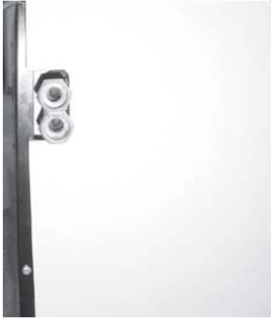
Attachment threading of the hot water heating element
