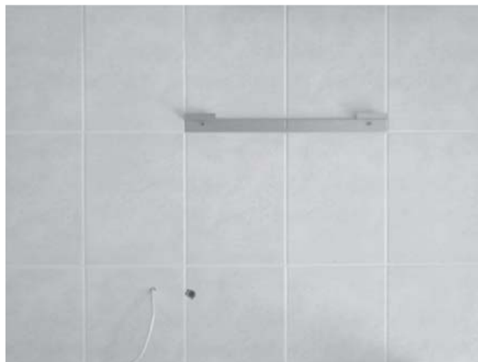
An example of preparation of electric power supply, condensate drainage and mounting of the bracket
