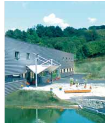
interscience R&D center and manufacturing plant
