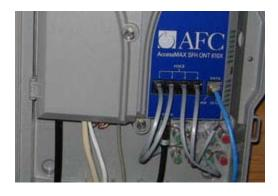
At left: An ONT with four (4) phone jacks. The model installed at your location will look similar but may not be identical to the picture shown here.
