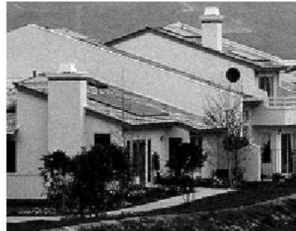
Individual Home Rooftop
