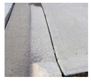
← Diamond Grinding and Diamond Sawing have the same effect on the Concrete surface, exposing the aggregate as clearly seen in these photographs.
