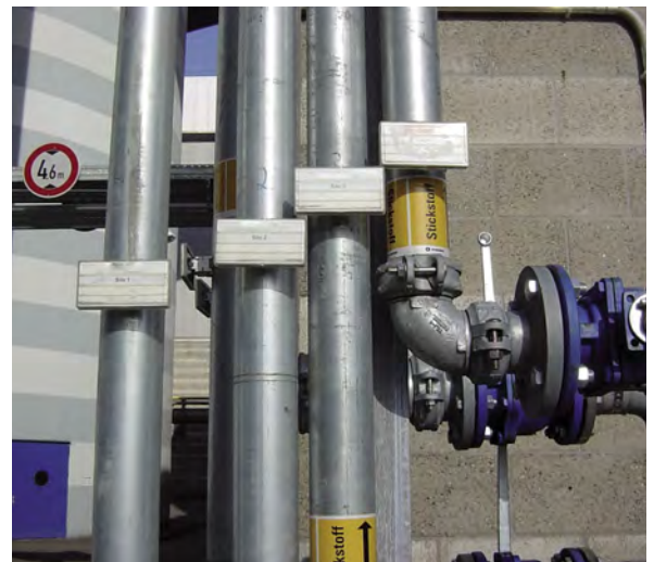
Picture 10: Inert gas feeding through pre-installed pipes
