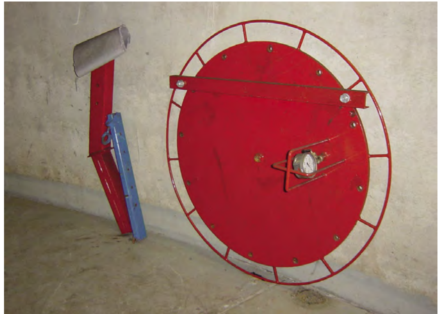
Picture 2: Prepared sealing for clearing-out of silo
