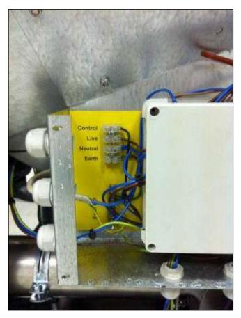
Brown - Time Clock Control Live Black – Permanent Live Blue – Neutral Green / Yellow – Earth Only authorized TR Engineering personnel may open the control panel on the boiler. Any interference with the wiring in the control panel will invalidate the warranty. The boiler and complete plumbing system must be adequately earthed and bonded in accordance with local Building Regulations and Bye- Laws.
