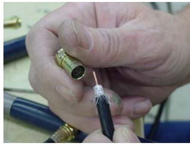
Attach Coax Connector to end of Coax Cable
