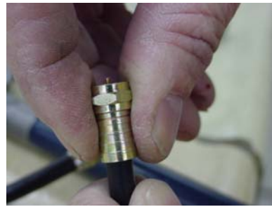
Attach Coax Connector to end of Coax Cable
