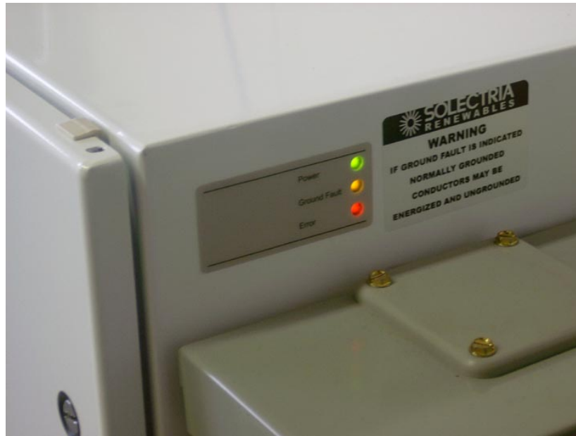
Fig. 8. The view from right-hand side of inverter above DC (PV) disconnect (LED indicator during initialization, all LEDs on)
