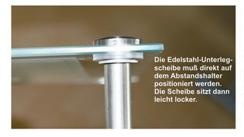
The stainless steel gommet have to be placed on the distance piece directly!
