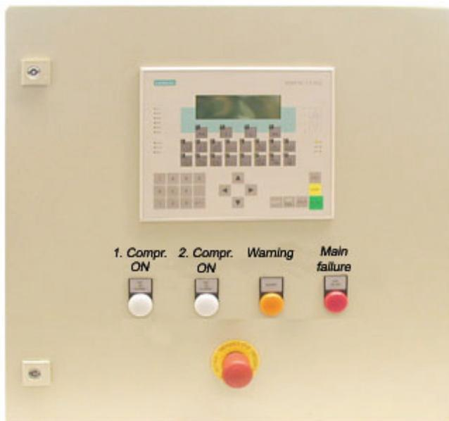
Figure 1.1: View of outside of switchgear cabinet
