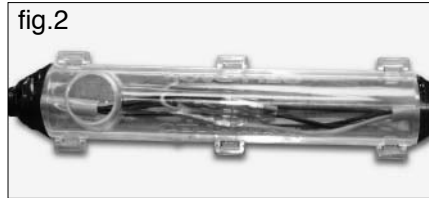
Fig. 2: Enclose connection in appropriate watertight enclosure and seal both sides
