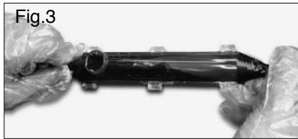
Fig. 3: Fill enclosure with plastic resin
