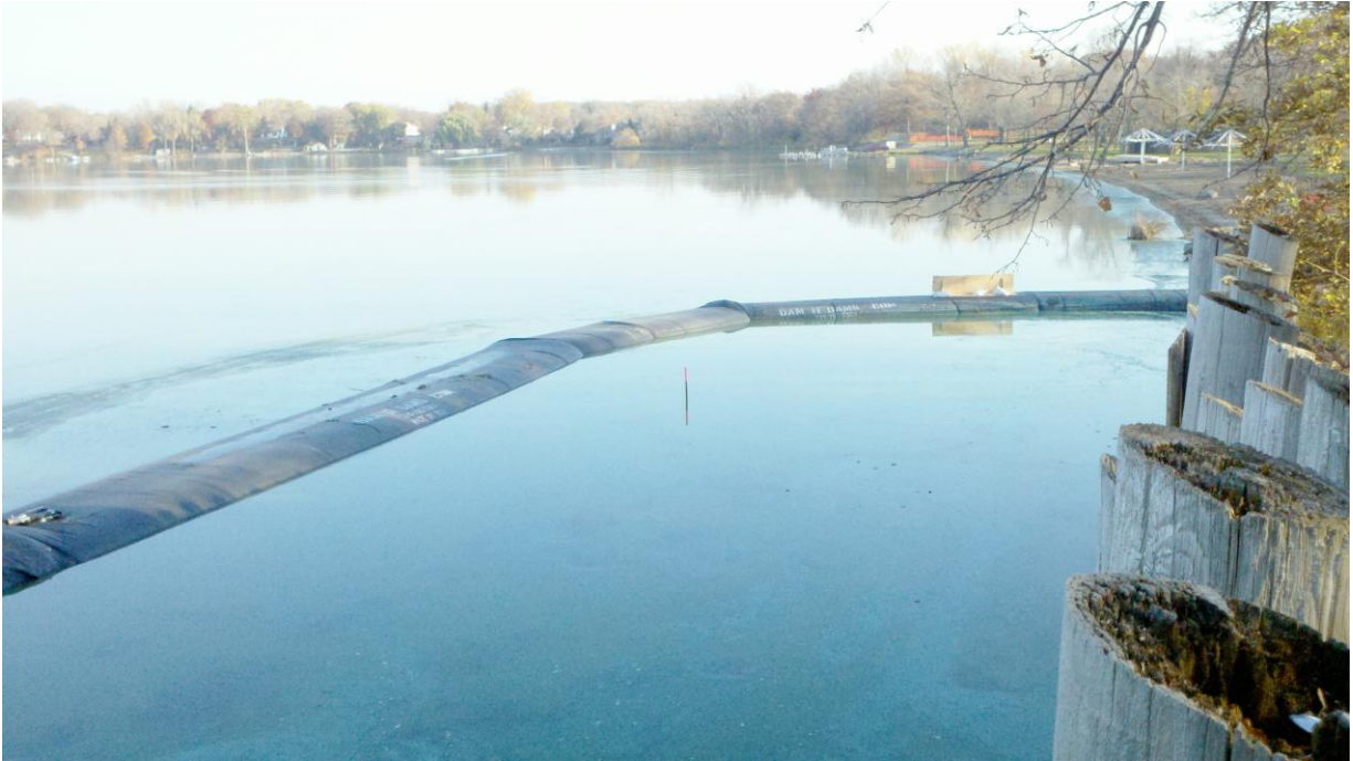
Figure 9 – A long cofferdam with coupling collar connections.
