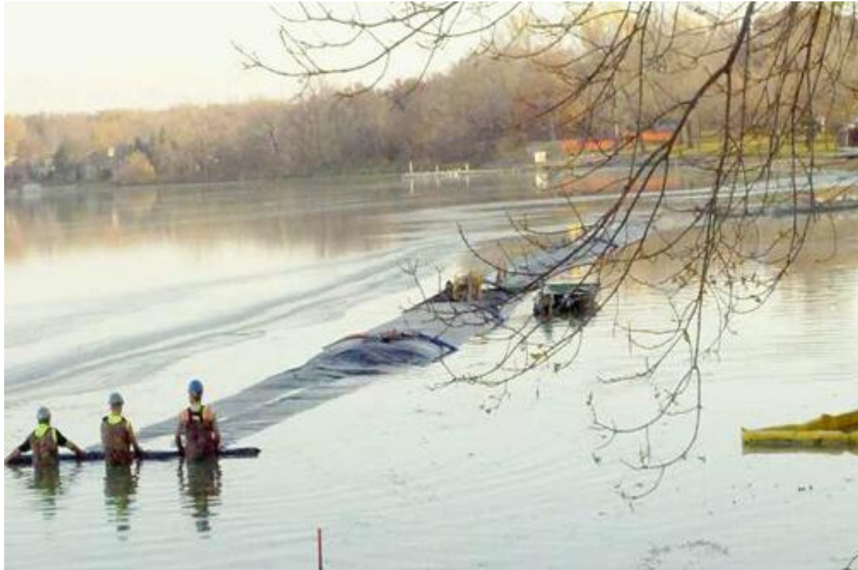
Figure 23 – Workers standing against rolled end of a cofferdam as it inflates.
