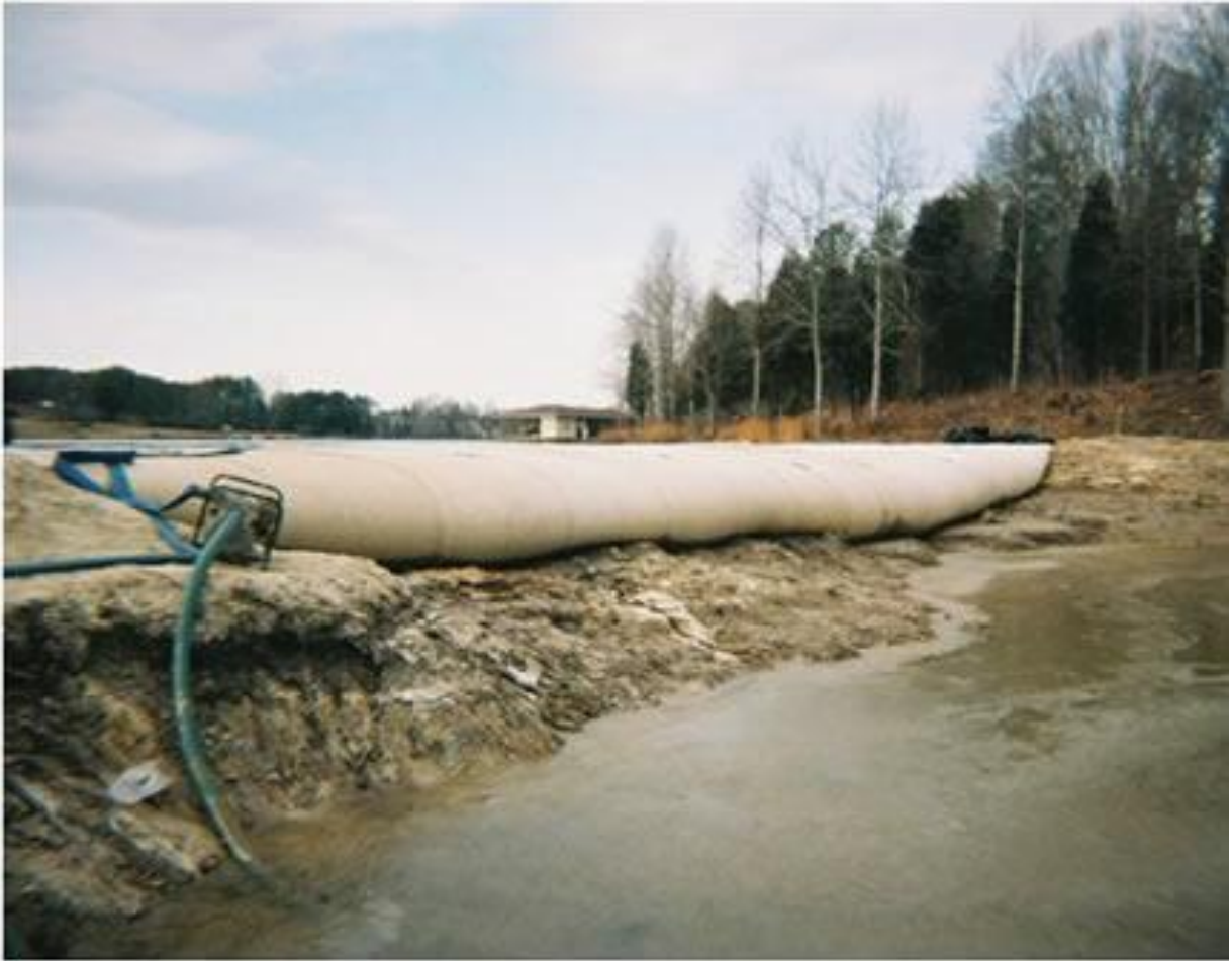
Figure 5 – Cofferdams mold to the environment to seal and prevent water escape.
