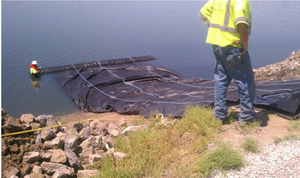
Figure 17 – A worker guides the cofferdam as it inflates and unrolls.
