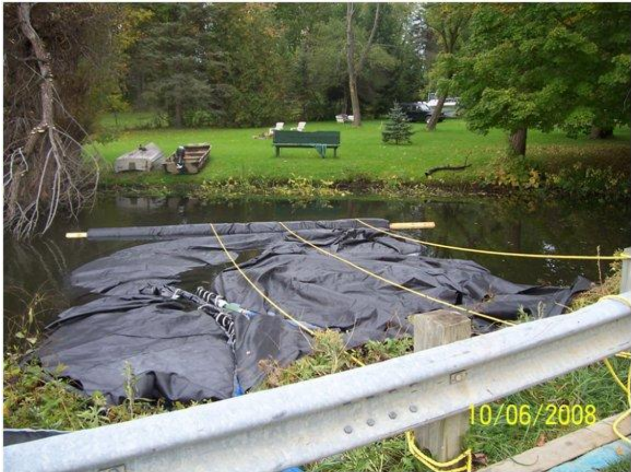
Figure 24 – Restraining ropes should be used to control large cofferdam installations.
