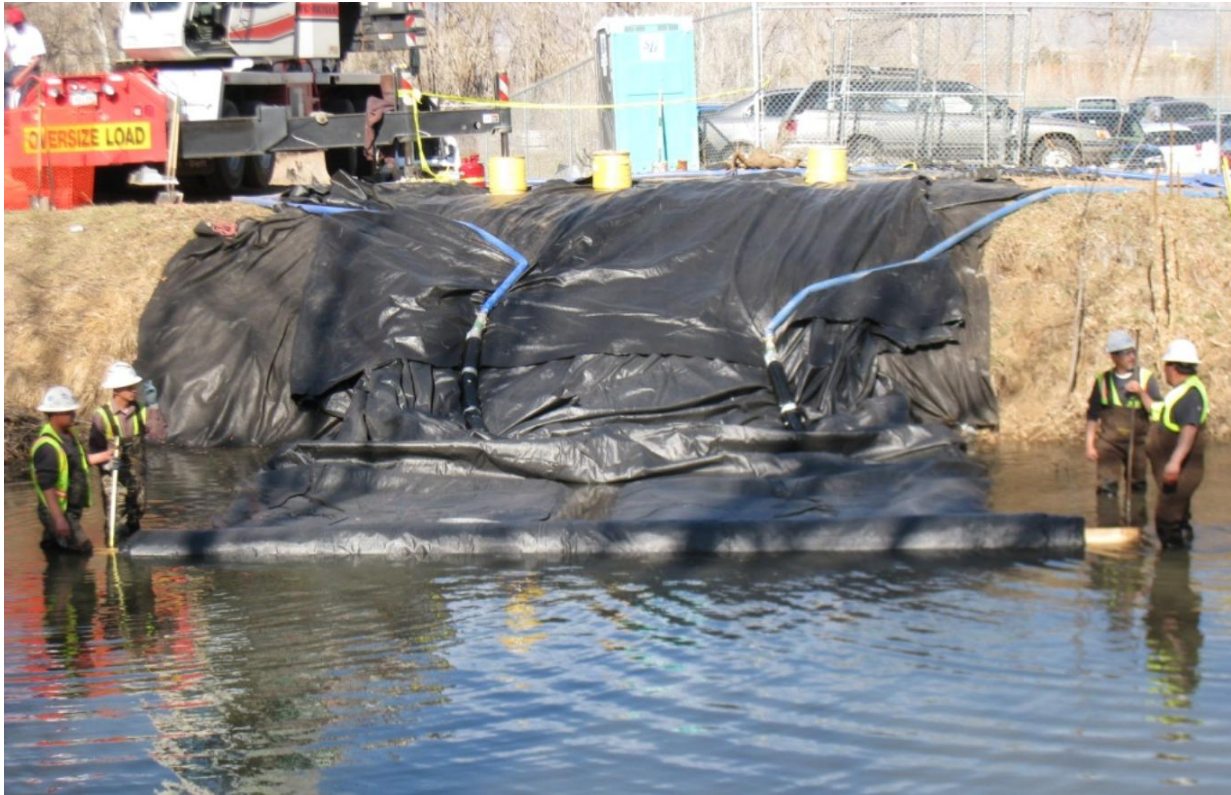
Figure 21 – Fill tubes are inserted into a cofferdam resting on a bank.
