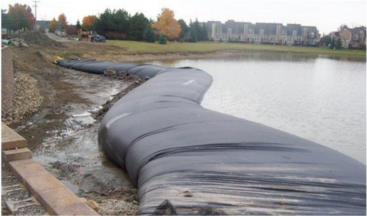
Figure 11 – Cofferdams can accommodate several different angles to keep water out.
