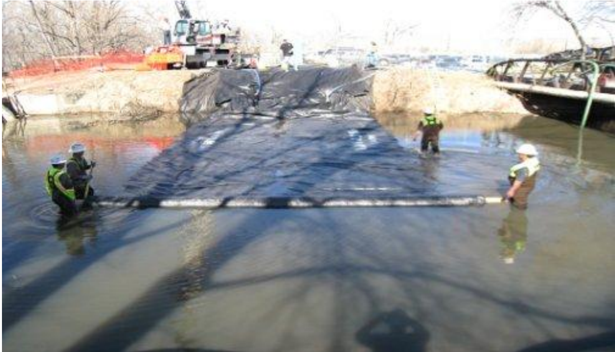
Figure 13 – Workers guide the unrolling of a large cofferdam as it inflates.
