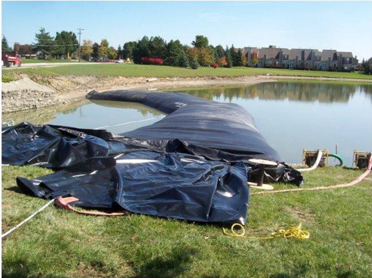
Figure 15 – Fill tubes carry water from the discharge pumps to inflate the cofferdam.
