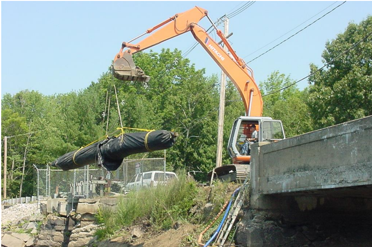
Figure 20 – A large cofferdam is delivered to the project site using loading straps.
