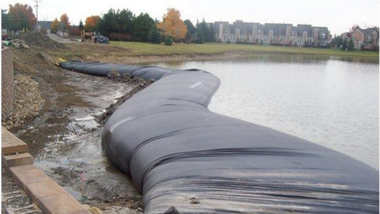
Figure 4 – Dam-It Dams’ cofferdams can withstand tremendous lateral pressure.
