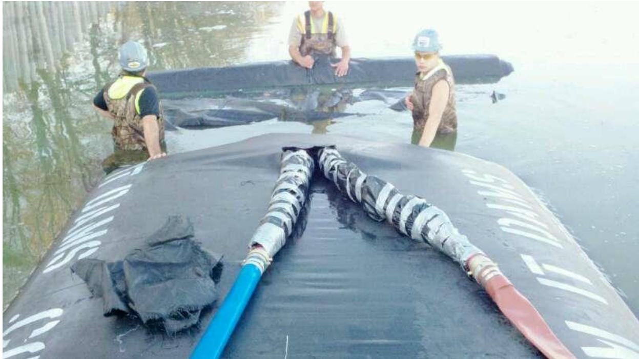
Figure 28 – Discharge hoses are fully inserted into inner fill tubes.
