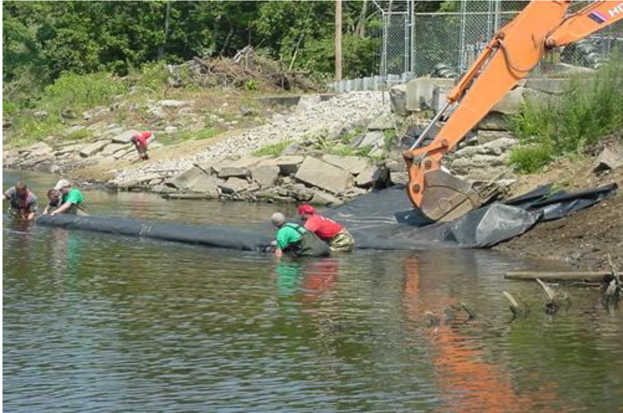
Figure 16 – A cofferdam is properly positioned at the Starting Point.
