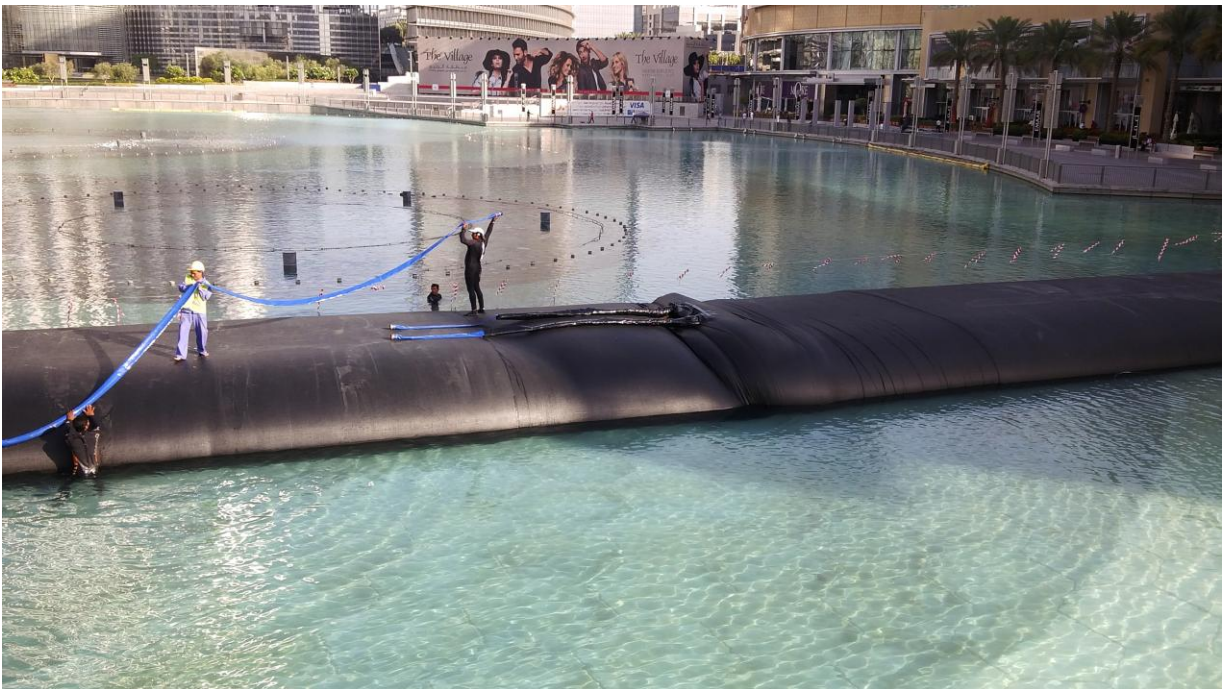
Figure 10 – Two cofferdams joined by a coupling collar.
