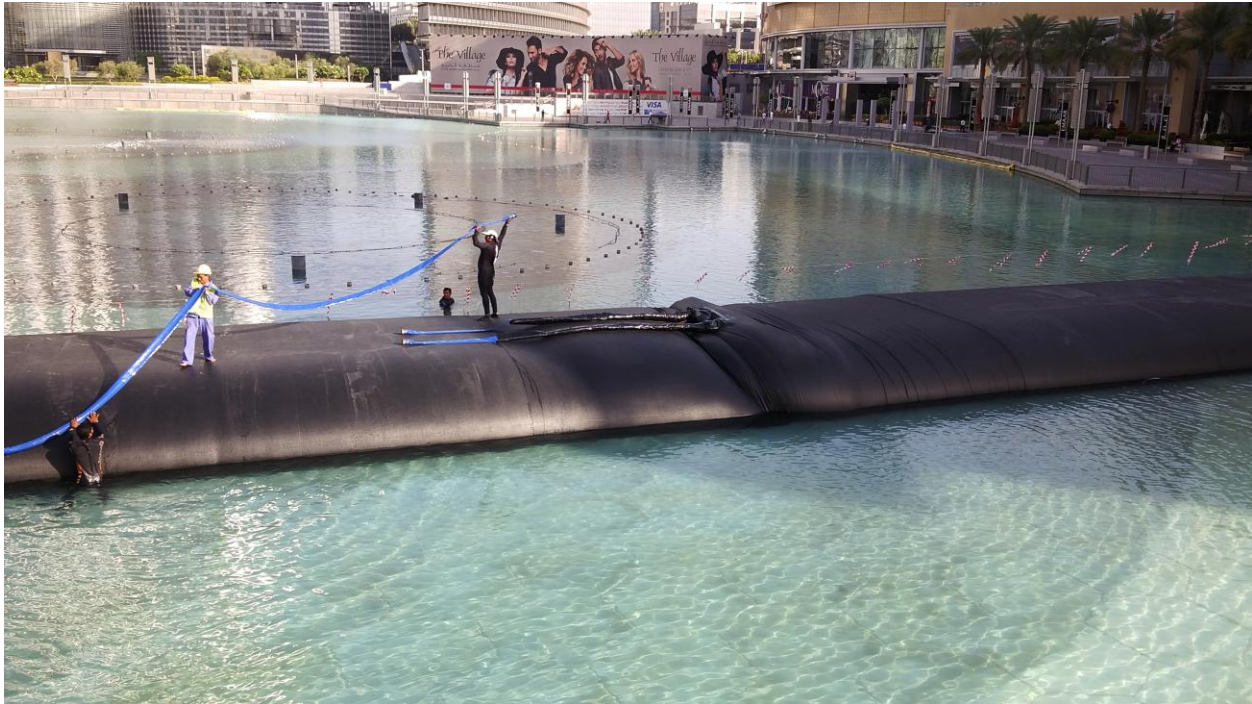
Figure 26 – Two cofferdams are connected with a coupling collar.
