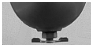
picture 7.3.4 drain valve on the water cutoff
