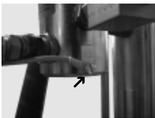
picture 2.4.1 ground screw on the high pressure filter
