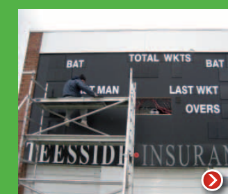
Fitting new fascia and components
