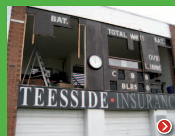
Removal of existing fascia and framework
