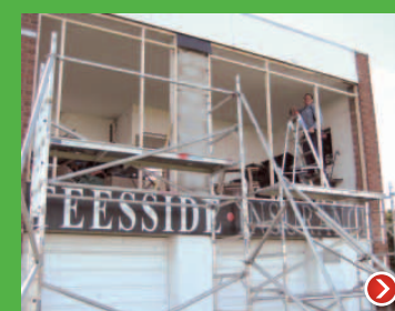
Construction of new timber framework
