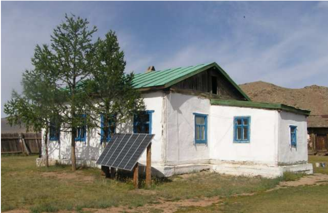
The PV array at the hospital of the Murun Bag
