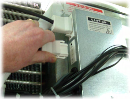
Figure 4: Connecting the Sign plug (SK500-3)
