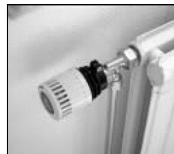
Open the thermostat valves completely.
