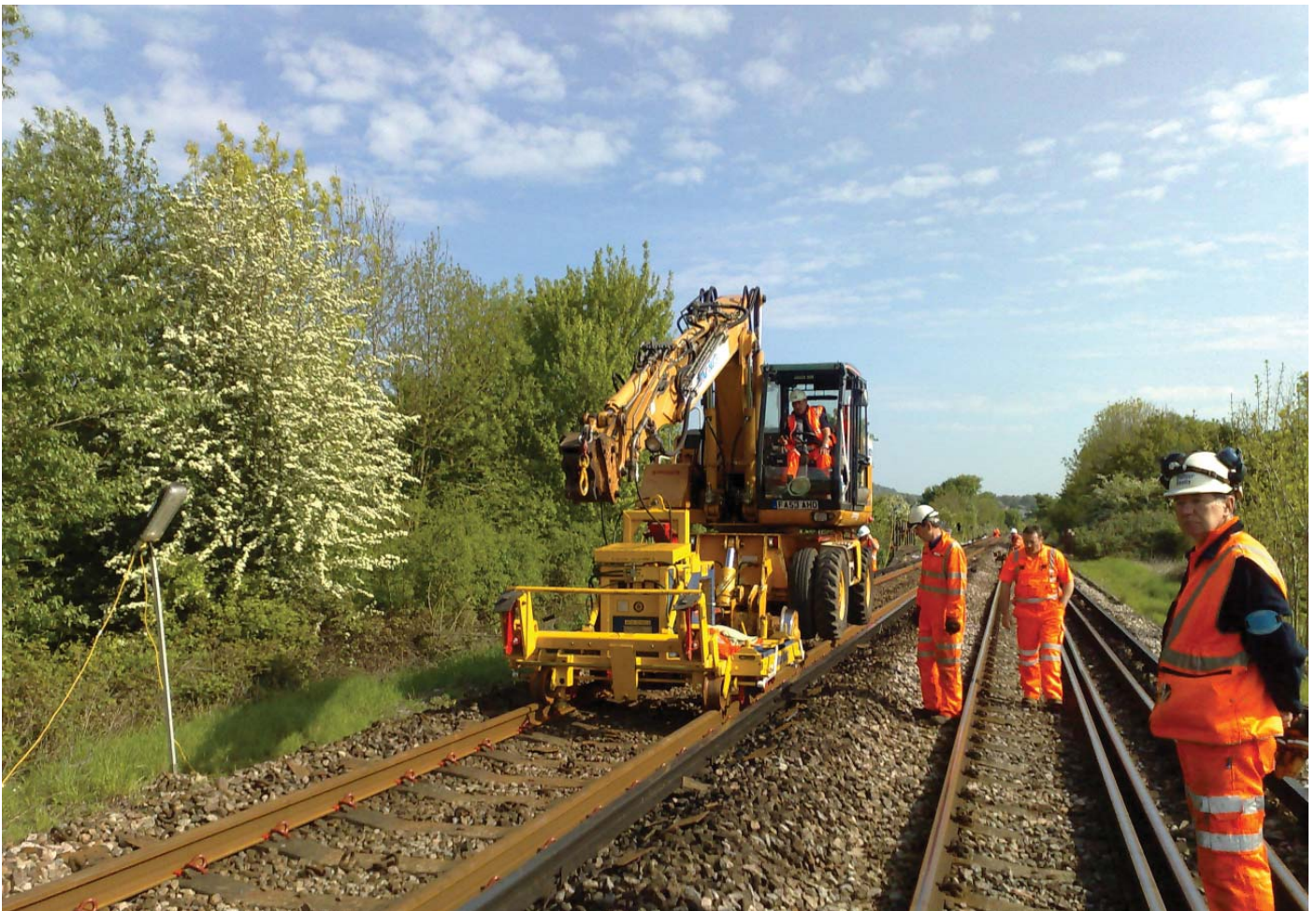
Fastening PR 401 Clips with the Thomson PR 401 clipper
