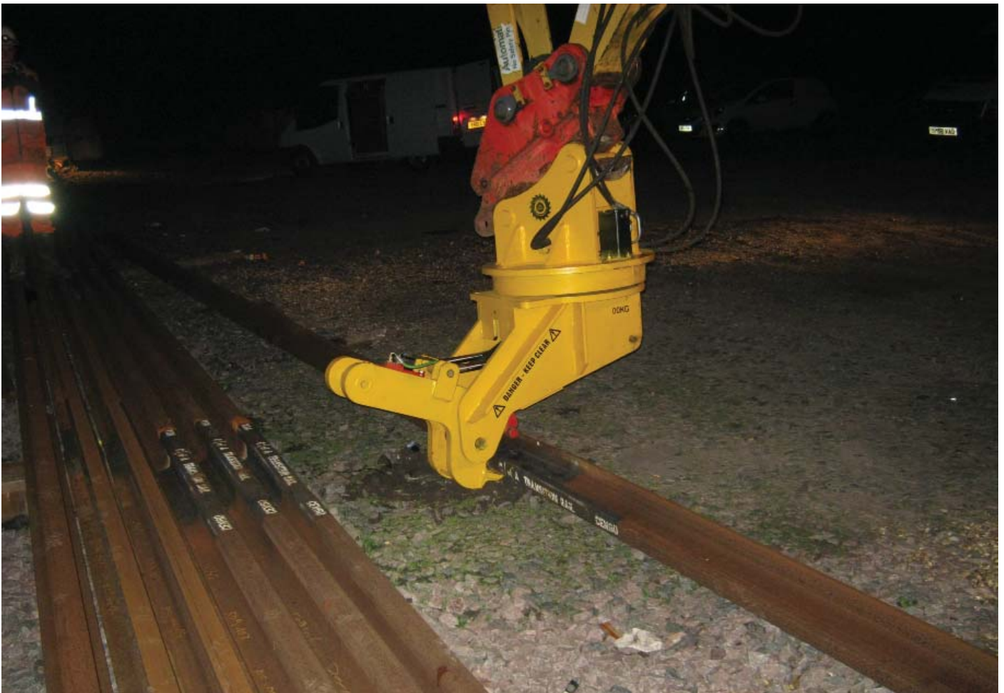
Recovering, Turning and Stacking Rails using the RT211 Cuttlefish Rail Turner
