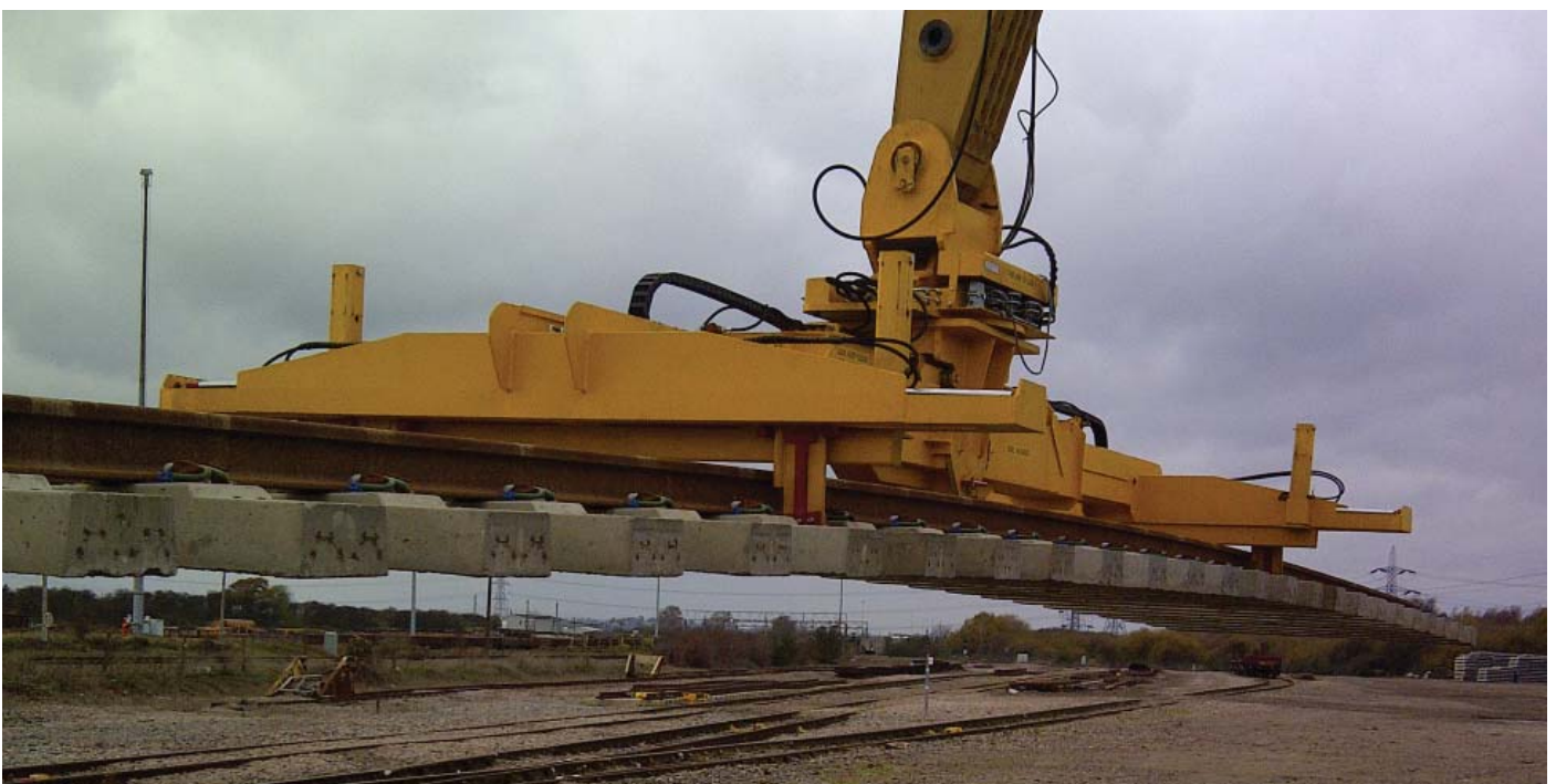
Loading an 18m Track Panel using a Thomson Megabeam
