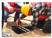
**Recording the Data** If there are specific details about the utility that need to be recorded, we recommend you create a standard form to write them on. Recording the data should be done while the hole is open. If you are digging several holes a day, recalling the details of one from another is tough. Some of the things you may want to write down are: size, depth, material, color, condition of utility, soil condition (type of fill,
