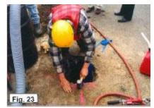
**Starting the Spot Hole** Although it is not necessary, you may want to start the test hole with a shovel, digging bar or other hand tool. This will reduce the amount of blowing dust and dirt once the air lance is inserted. If working around fiber optic cables, gas lines or PVC piping, extreme care must be taken when using hand tools. Keep the opening in the ground as small as possible. We recommend an initial cut of 8"x 8". After the hole has been started, use the air lance to pinpoint the
