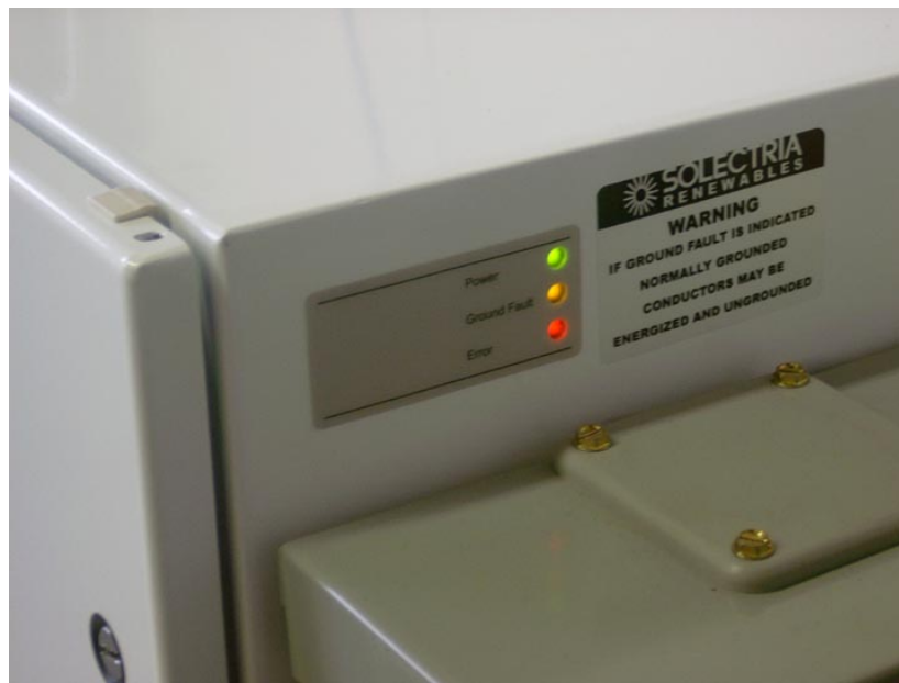
Fig. 8. The view from right-hand side of inverter above DC (PV) disconnect (LED indicator during initialization, all LEDs on)
