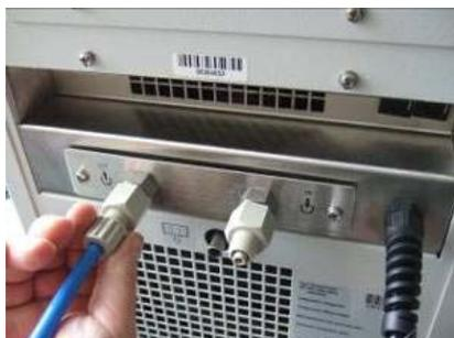
7. Repeat this procedure to connect the second coolant hose from the evaporator **coolant out** connector to the re-circulating cooler **return** (or **in**) connector.
