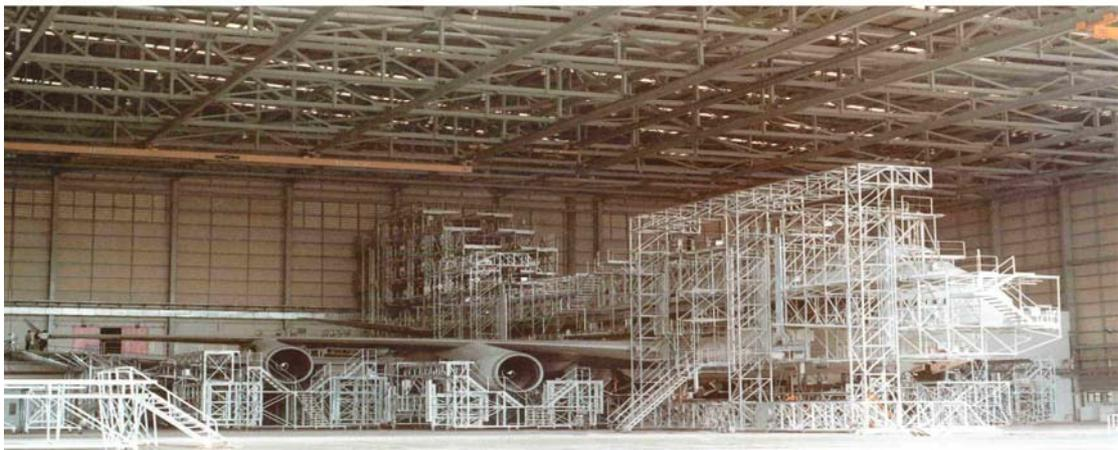
Figure 2.1. Fixed Working Platforms
