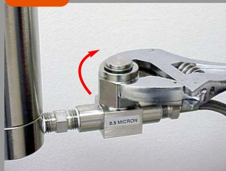
Use wrench, tighten the T-filter cap firmly. Open LCO<sub>2</sub> tank valve and check for leaks.
