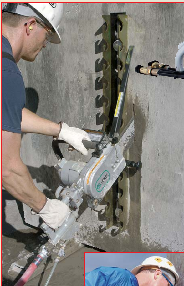
Above: Optional SpeedHook® guides saw for straight cutting.
