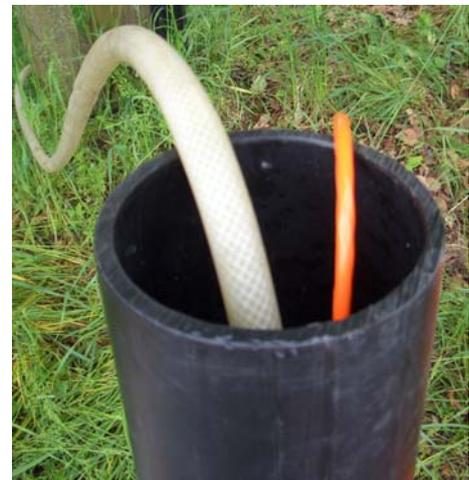
16. Terminate the installation as specified. It is important to terminate the cable above ground level in a waterproof enclosure or with a waterproof connector. Protect the installation from construction traffic and mark its location with a stake.
