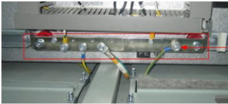
Figure 4-4-5 PE copper in the inverter
