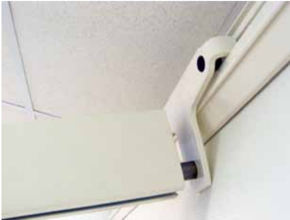
Figure 65. Fitting of traverse rail to telescope trolley and fixed trolley
