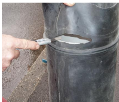
Photo 2.2.3 (5): distance of EPDM rubber from sleeve edge
