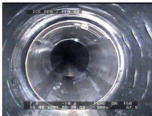
fig. 2.3.9 (2): drain pipe after repair
