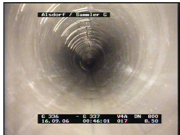
fig. 2.3.3.(4): photo A finished serial installation. All locks in row
