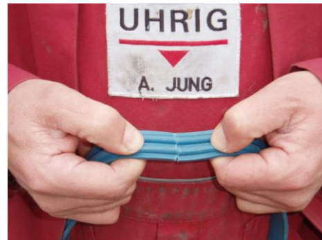
fig. 2.3.6 (2): join the ends of the swelling rubber with super glue
