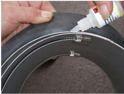
fig.2.2.4 (6): fix EPDM rubber
