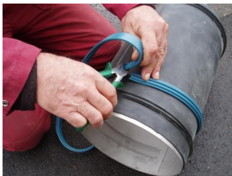
fig. 2.3.6 (1): Cut the Swelling Rubber to the correct length
