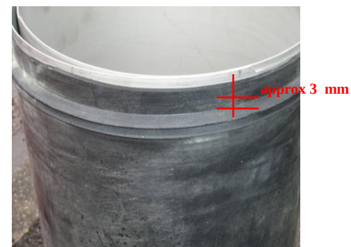
Photo2.2.4 (4): EPDM rubber. Cut overlap
