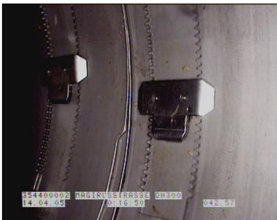
fig. 2.3.3 (3): photo Sleeve overlaps Sleeve in Sleeve
