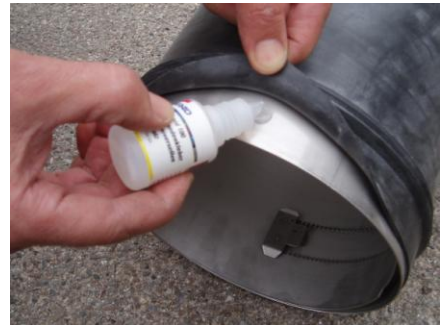
fig.2.2.4 (7): fix EPDM rubber
