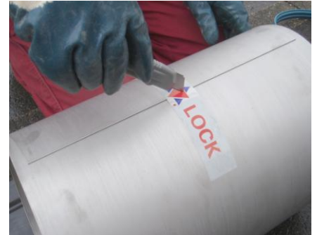
fig. 2.2.4 (1): cut adhesive strip only halfway through
