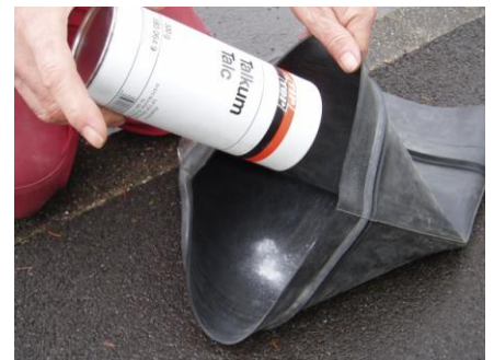
Photo. 2.2.4 (2): Sprinkle Talc inside EPDM rubber
