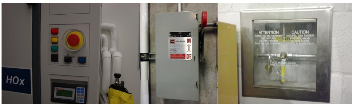
Figure 5.3.2-1: Examples of electrical and gas shut-offs
