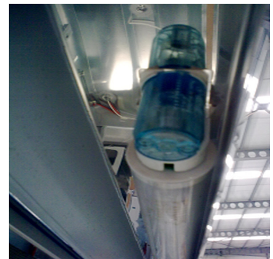
The starter is located adjacent to the tube
