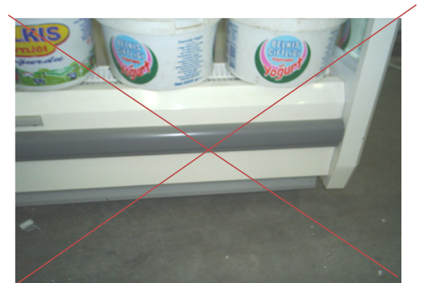
Never place somethings in a position which may restrict air flow
