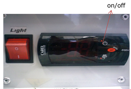
Power button to turn on&off the case Warning: This will not isolate the case!
