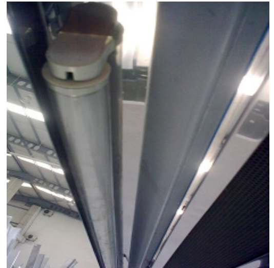
The lighting tube is located in the case canopy
