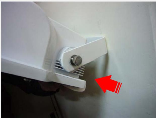
5. Attach the two M10 screws to both sides, adjust the irradiation angle of the luminaire, and tighten the screws on both sides.
